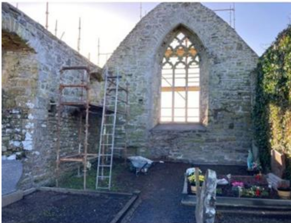
TRACERY WINDOW, ST KERRILLS BEFORE AND AFTER WORKS 2022
