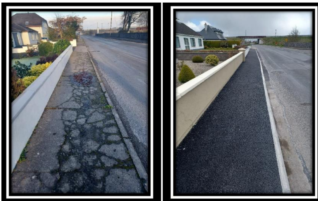
FOOTPATH REPAIR UNDER ACTIVE TRAVEL, WEIR ROAD - BEFORE AND AFTER
