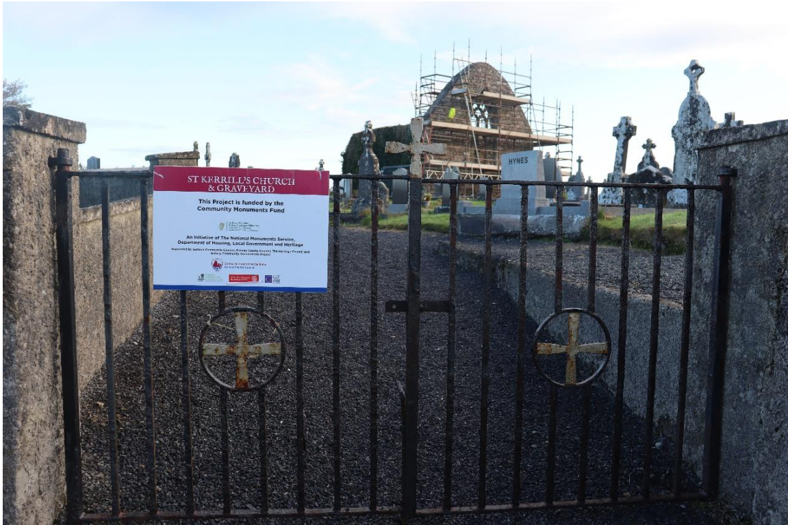
WORK IN PROGRESS AT ST KERRILLS ABBEY, CLOONKEENKERRILL, GURTEEN.
