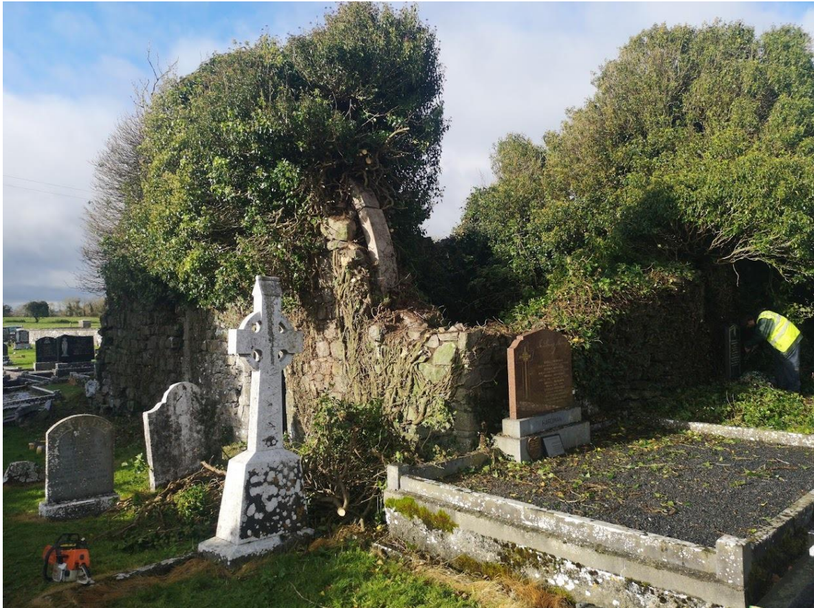
ABBEYGORMICAN TRANSEPT CHAPEL AND HANNON TOMB DURING CLEARANCE WORKS
