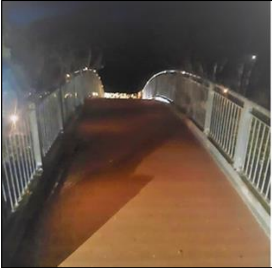
LED STRIP LIGHTS ON HANDRAIL
