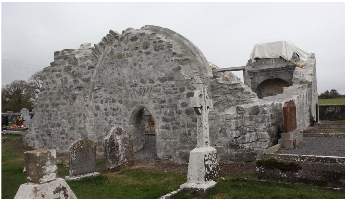
ABBEYGORMICAN TRANSEPT CHAPEL & HANNON TOMB AFTER CAPITAL WORKS 2021 & 2022
